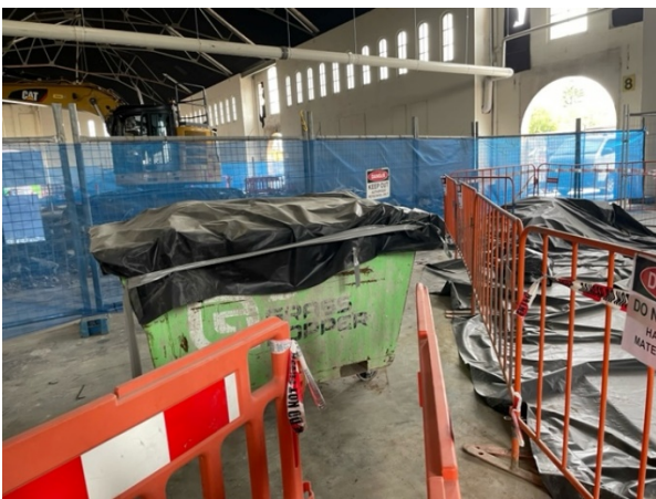
Separation and covering of potential Asbestos material
