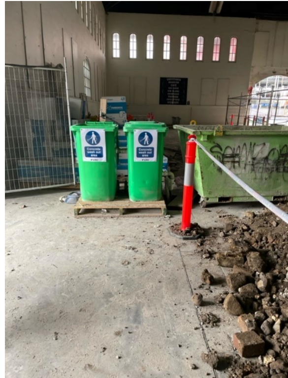
Concrete washout bins for hand tools
